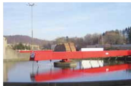
Enduring waste water cleaning helps to protect resources and results in cheaper production processes.
